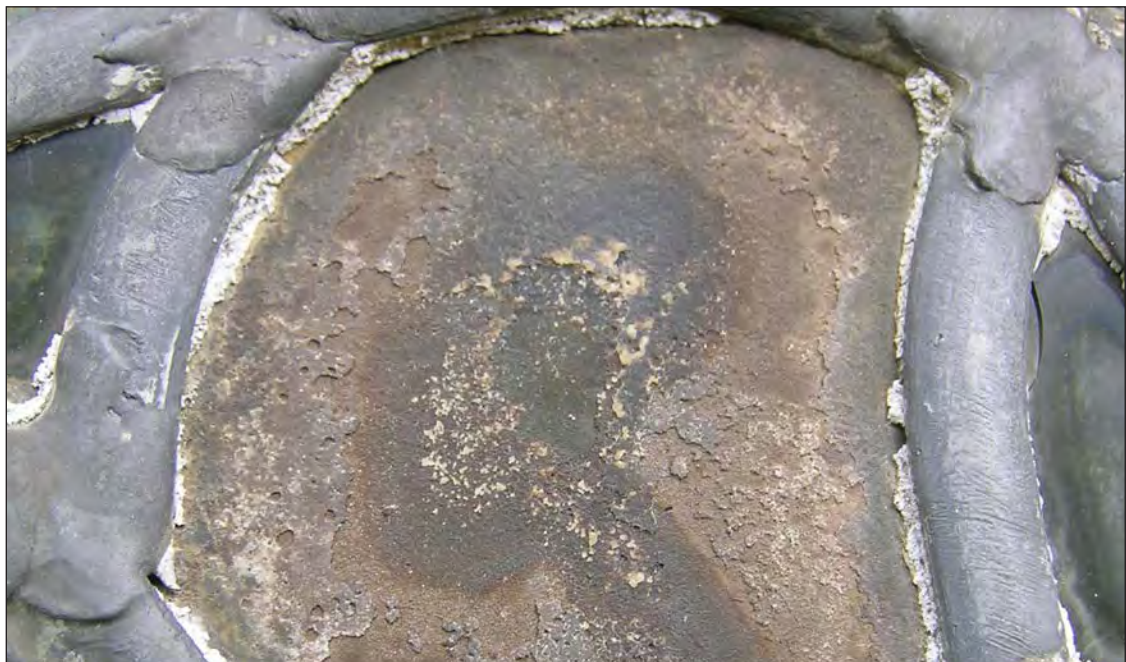
Figure 11. Weathering crust on the external surface of glass at Canterbury Cathedral.
