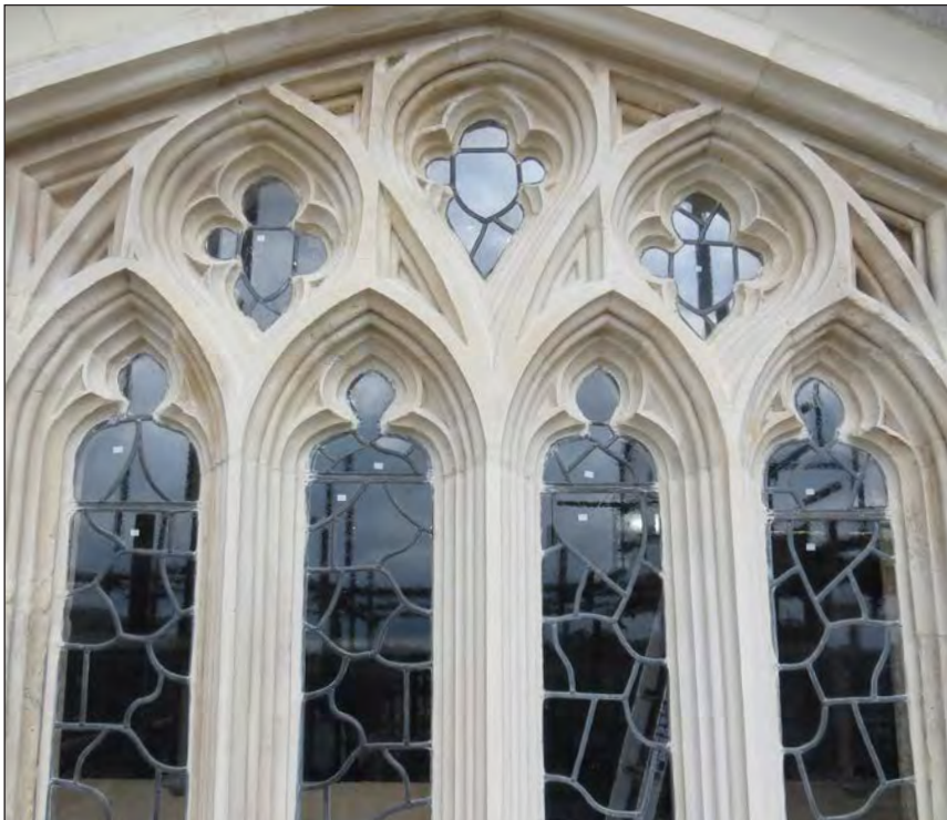
Figures 58, 59. Bad example (top) where the protective glazing covers parts of the stonework; and a good example (bottom) where the protective glazing is fitted into it.
