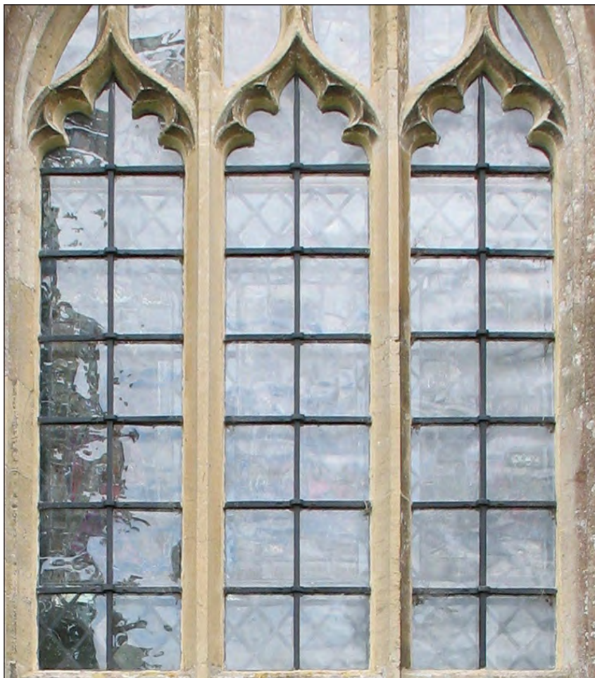
Figure 56. Chartres Cathedral, kiln-formed sheets slumped on moulds. ©Debitus Figure 57. Long Melford, kiln-distorted glass pieces cut to coincide with ferramenta bars.
