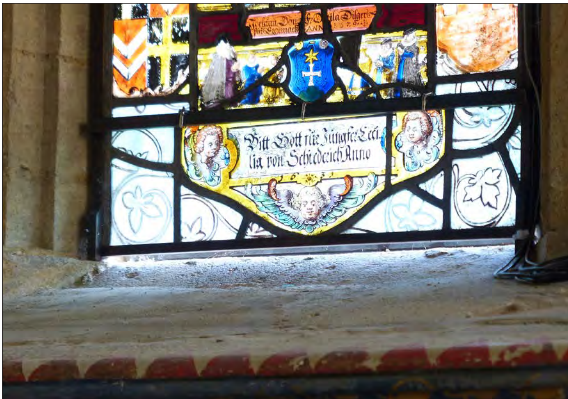
Figure 26. Internal ventilation openings at the bottom of the east window of St Andrew's Church, Trent, in Dorset.
