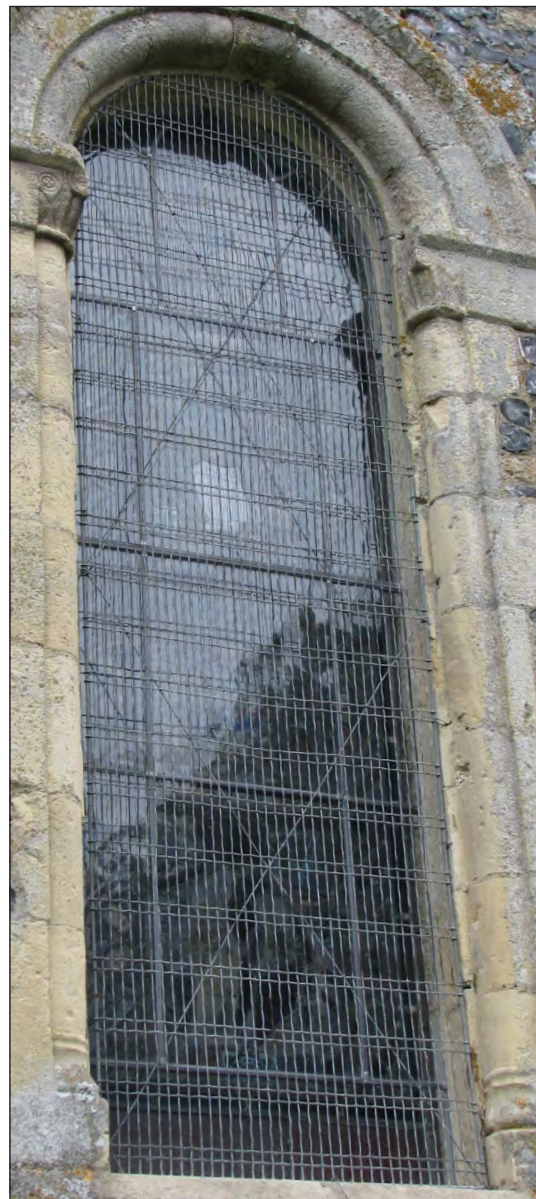
Figure 53. Cologne Cathedral, Schott low reflective glass. ©Léonie Seliger Figure 54. Patixbourne, large pieces of mouth-blown glass in combination with wire guards. ©Léonie Seliger
