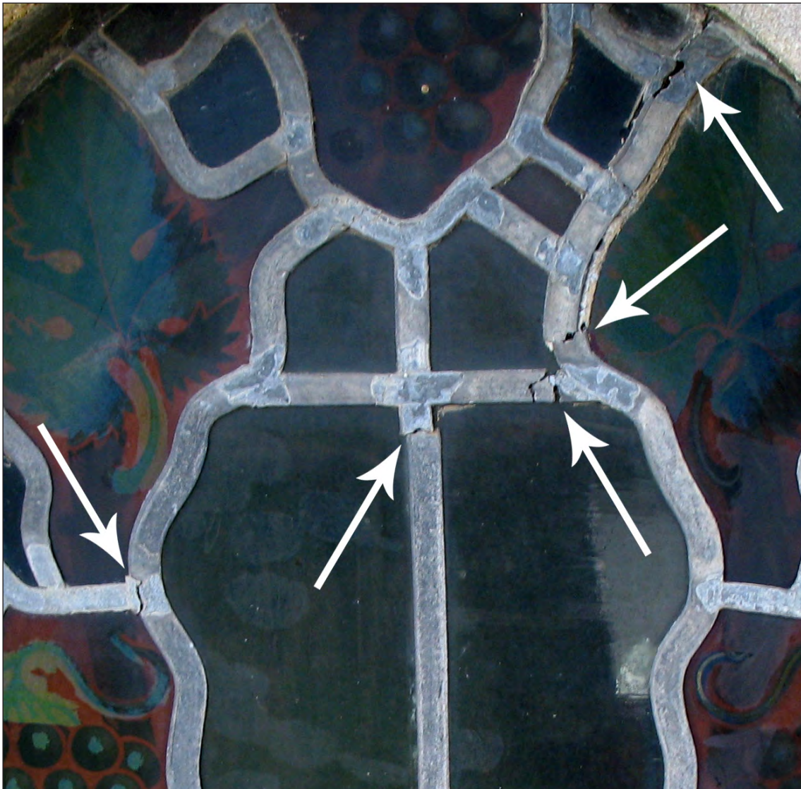
Figure 21. Fracturing of lead comes at vulnerable junctions. ©Léonie Seliger
