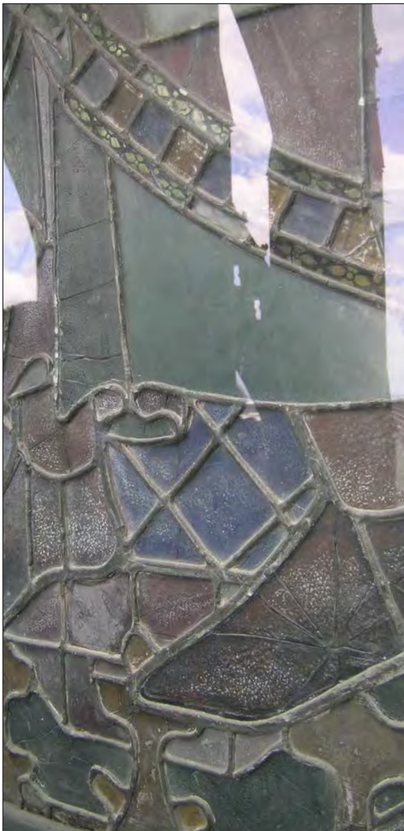
Figure 53. Cologne Cathedral, Schott low reflective glass. ©Léonie Seliger Figure 54. Patixbourne, large pieces of mouth-blown glass in combination with wire guards. ©Léonie Seliger
