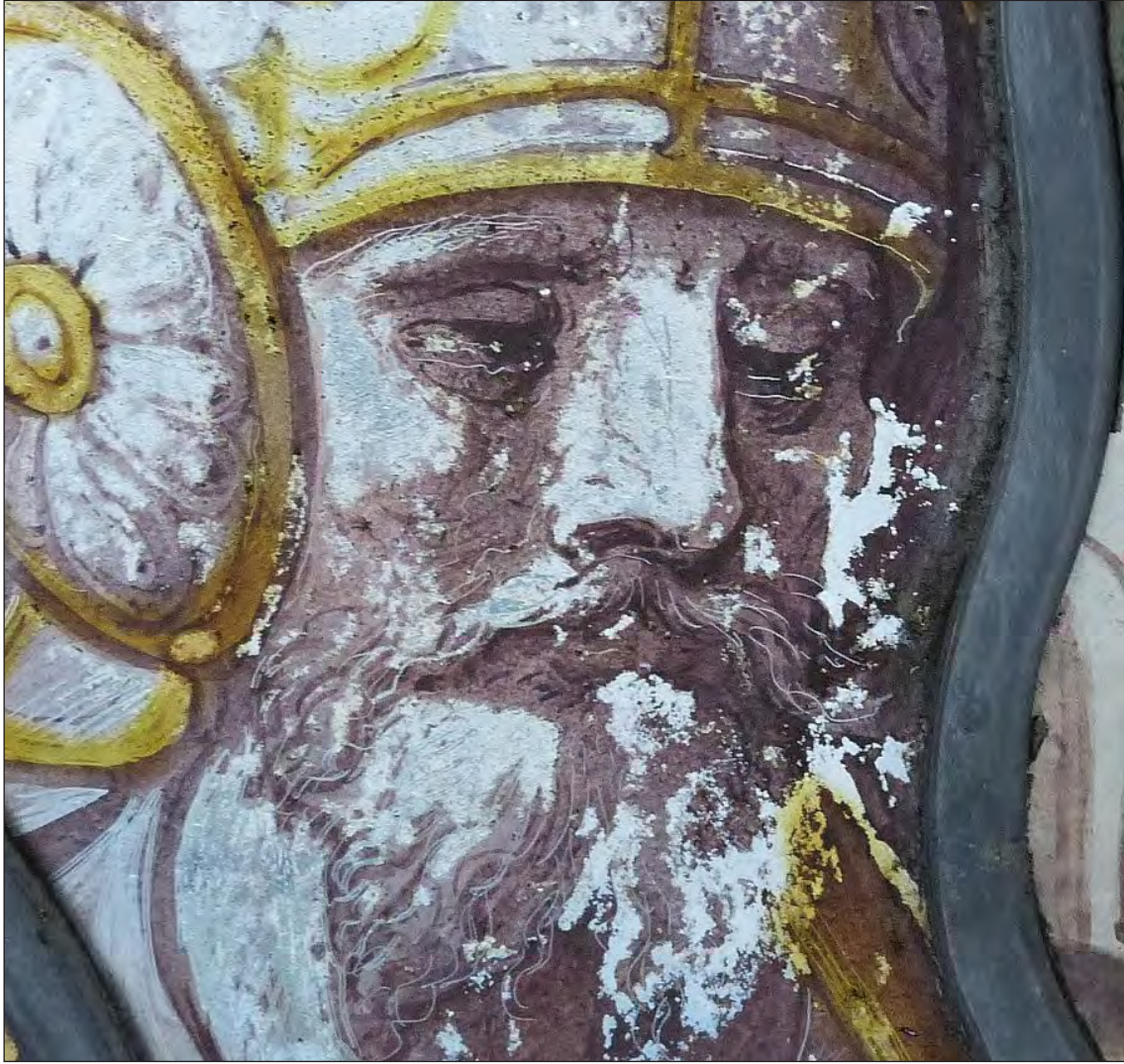
Figure 10. Loss of grisaille details on 16th-century glass at The Vyne.
