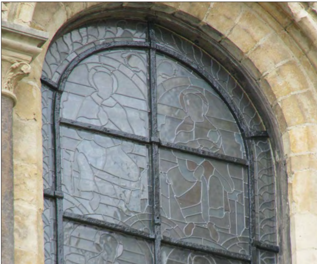
Figure 55. Canterbury Cathedral, kiln-distorted glass, leaded and given a thin coating of glass paint. ©Léonie Seliger
