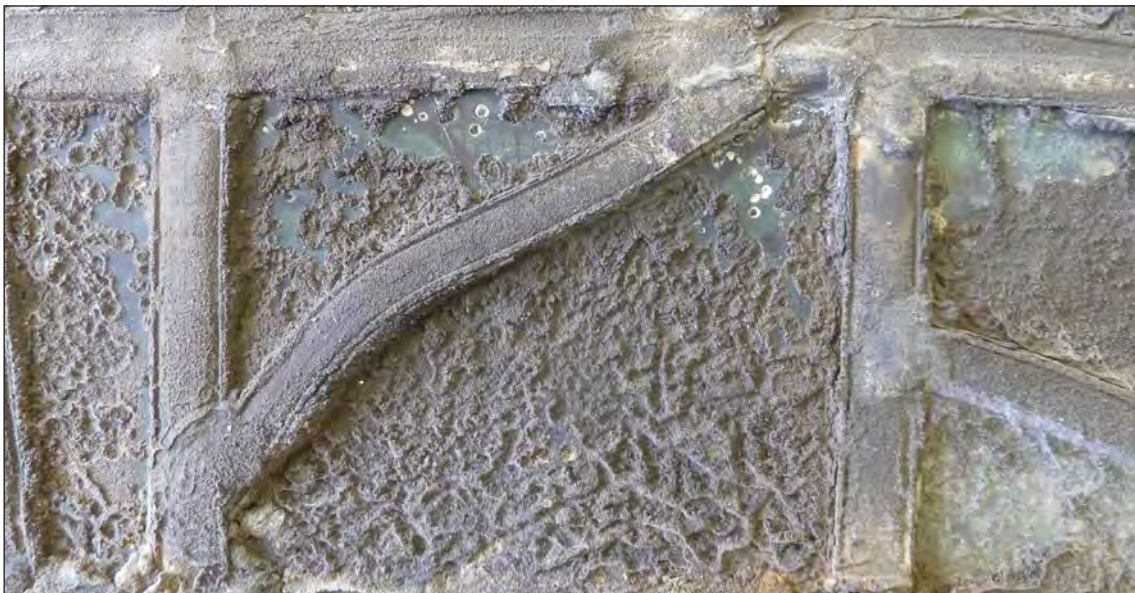
Figure 16. Pollutants accumulating on the external surface of historic glazing at Lincoln Cathedral.
