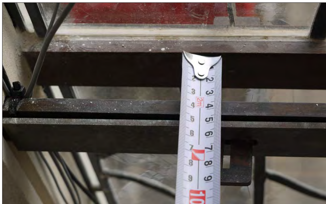
Figure 28. Interspace gap (before the reinstallation of the historic glazing).
