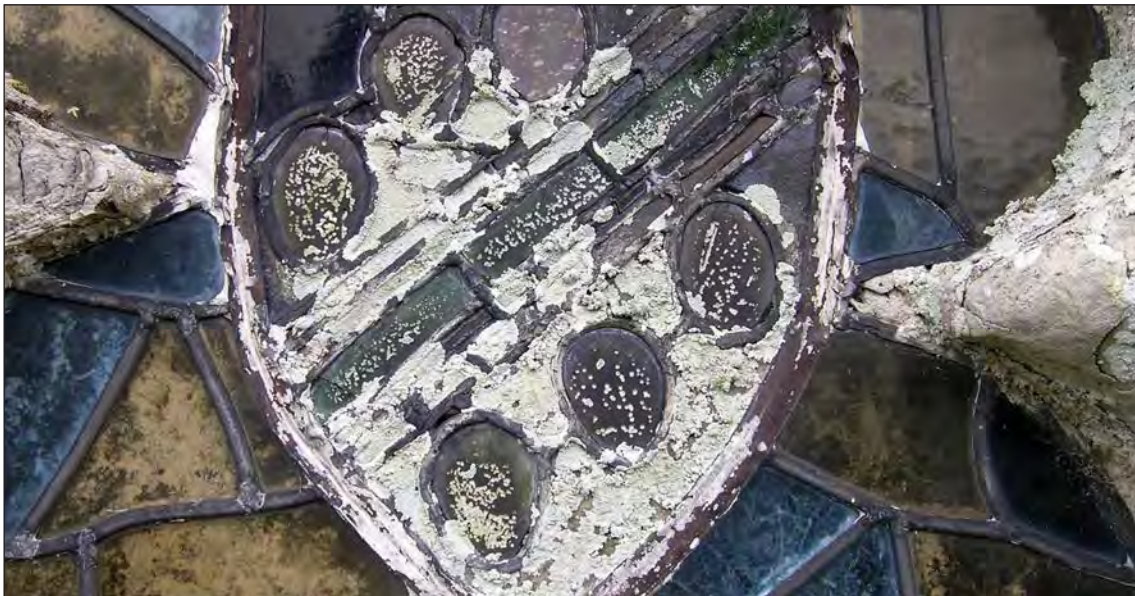
Figures 17, 18. Microbiological attack is both unsightly and can cause chemical deterioration of the glass as well as retaining moisture. Damage can occur internally as at Norbury in Derbyshire (top) or externally as at Boughton Aluph in Kent (bottom, ©Léonie Seliger).
