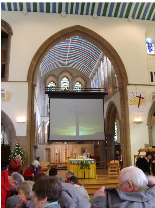
Large rear projection screen suspended in chancel arch. Note projector just visible above altar hanging. Screen is retracted above arch by remote control.
