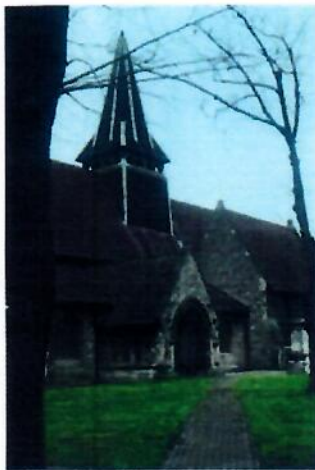
South Porch Entrance
